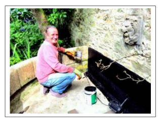
Jeff and I are also in the process of repairing the pond against the library wall. It has been cleaned out thoroughly again, bitumen mastic has been pushed into all the cracks we can find, and Jeff has been busy sealing the inside surfaces with bitumen paint – several coats will be needed. The library walls, like most of the stone used in buildings around the town, is the easily fragmented sedimentary sandstone called Cornish shillet, which can be very porous when
