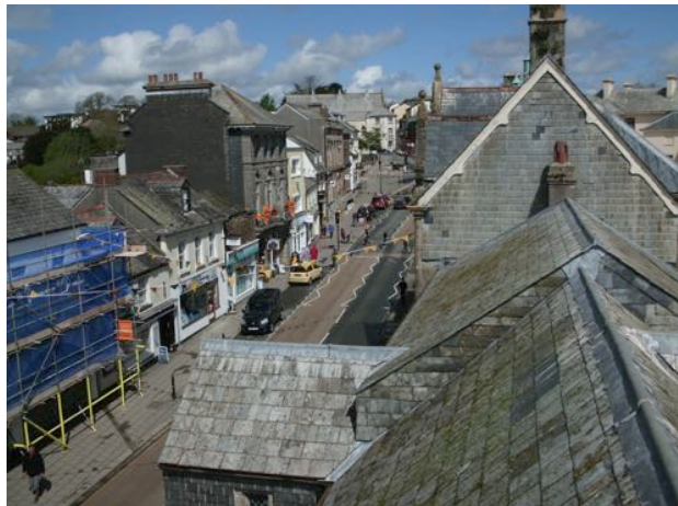
Roofscape 2015 – still lasting after another 20 years.
